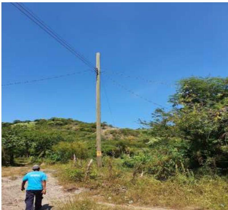
Source: Field visit, November 2019
