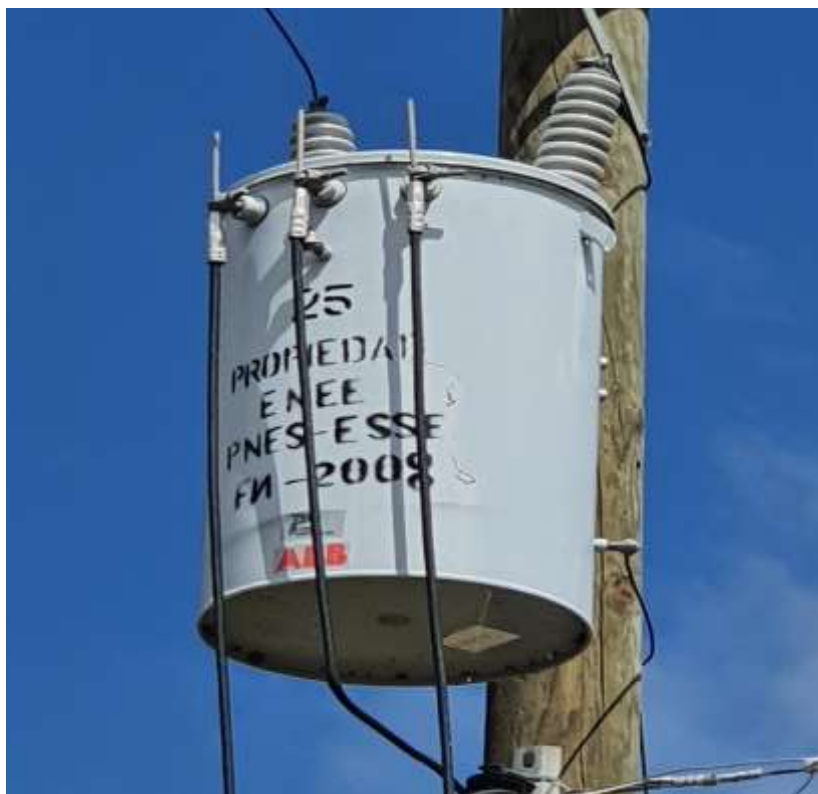
Source: Field visit, November 2019
